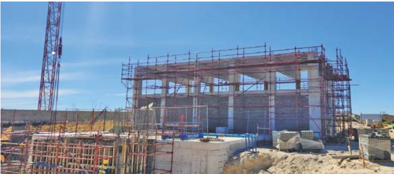
Gordon's Bay pump station's getting there: Construction of the Gordon's Bay sewer pump station and rising main is roughly 80% complete. The City is aiming for full completion by June.
